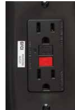
Typical GFCI receptacle
