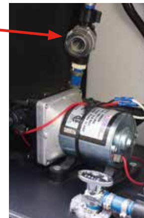
Typical water pump installation
